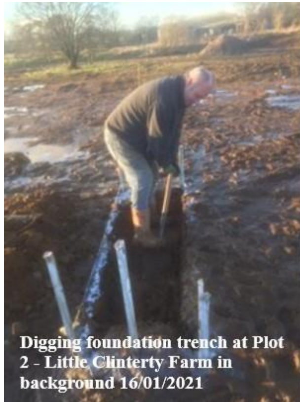
(Figure 4 - Commencement of Development – Foundation Trench Plot 2 – Burnside, Little Clinterty)
