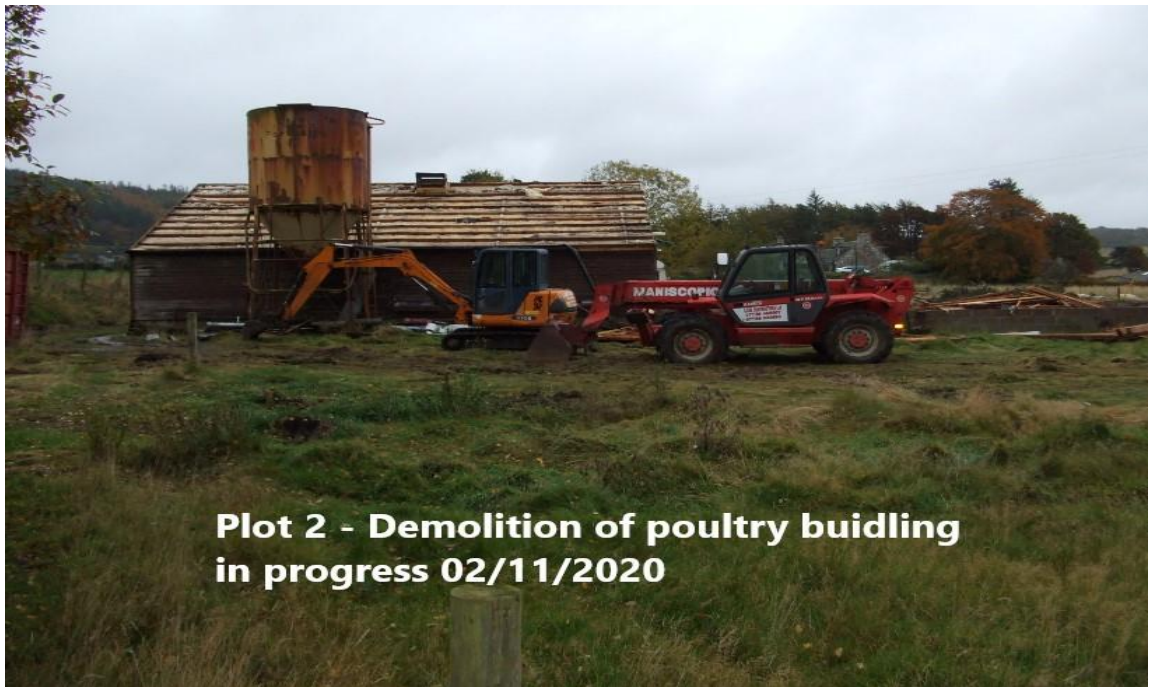
(Figure 2 Demolition in Progress – Plot 2 - Burnside, Little Clinterty)
